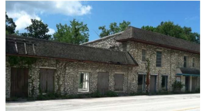
Existing structure/asset in AA-5
