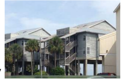
Figure 3.25: Buildings on pilings
