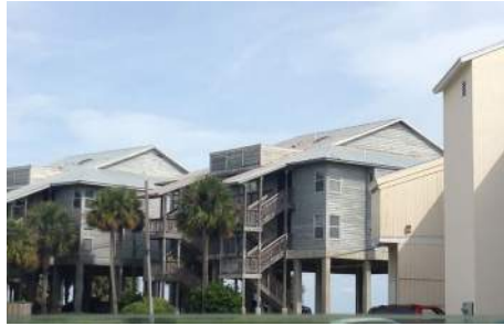
Figure 1.5: Houses elevated on pilings
