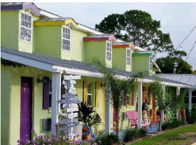
Figure 4.32: Low Key Hideaway motel an RV resort in CK
