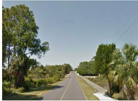
Figure 3.10: Street view of Area B
