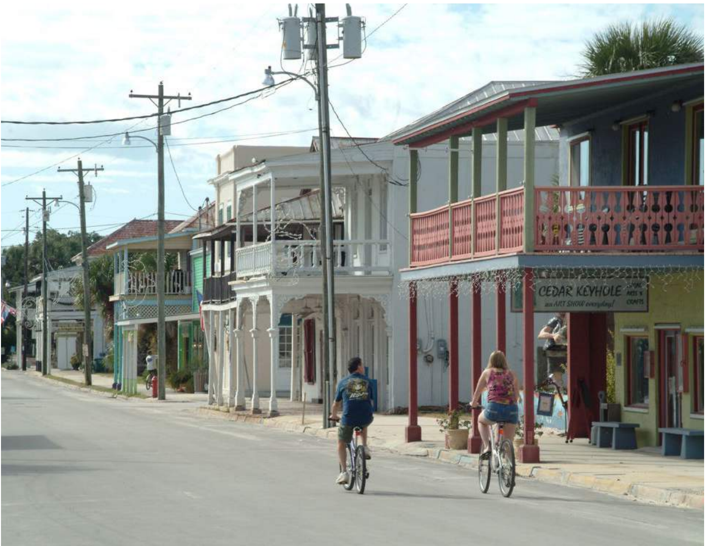
Figure 4.26: Downtown Cedar Key buildings have shaded walk ways which enhance the pedestrian experience
